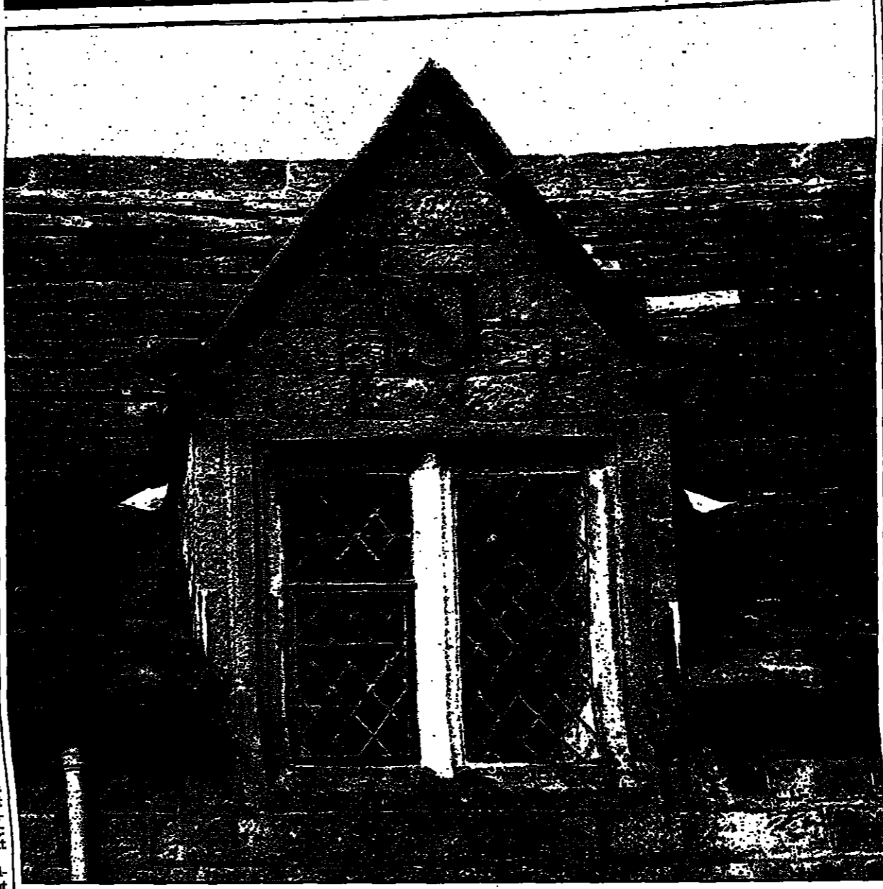
A traditional stone roof in Derbyshire, of the type English Heritage wants to restore and promote PHOTOGRAPH: DON MCFARLANE
